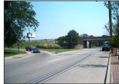
Pedestrian Safety Issues at I-64 and Story Avenue
