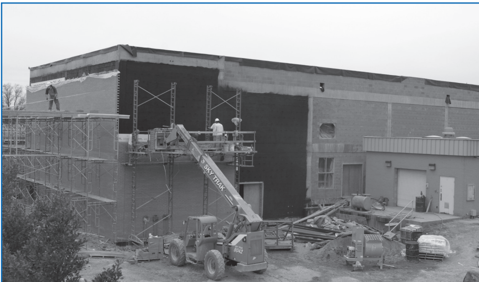
Construction of the On-Site Chlorine Generation Facility.
