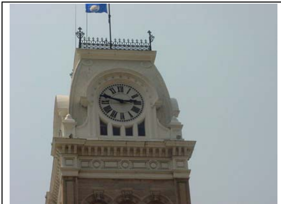
Clock Tower Renovation
