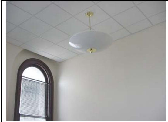
Office Renovation - Ceiling and Light Fixture
