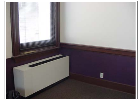
Office Renovation - Paint and Wall Air Unit
