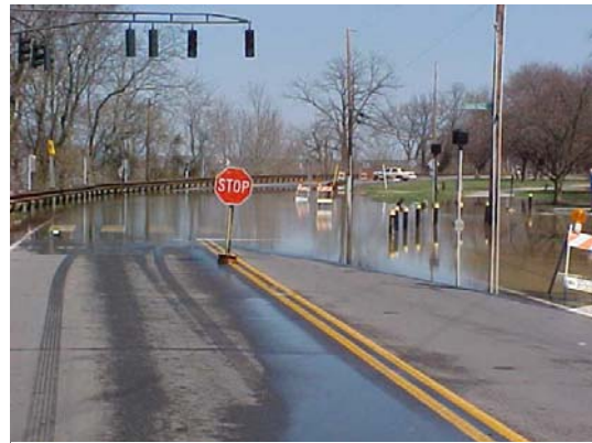
Figure 6. 2008 Flooding along River Road
