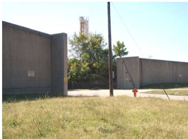
Floodwall at 11 th Street
